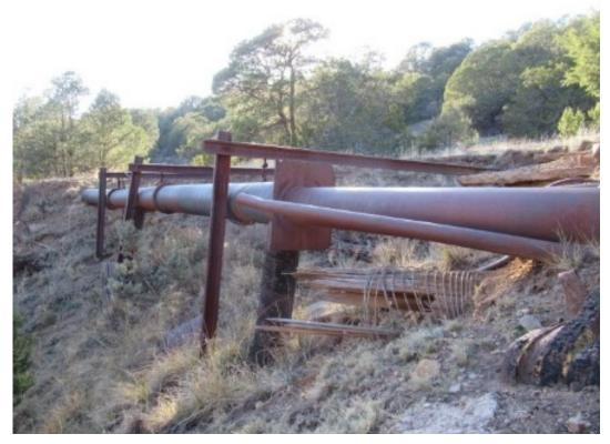
Here is a closer look. The replacement transite pipe (above) and older wooden pipe (wrapped with flat metal bands) - the material of our barns. The oak stays were removed and used as siding, floors and interior walls.
