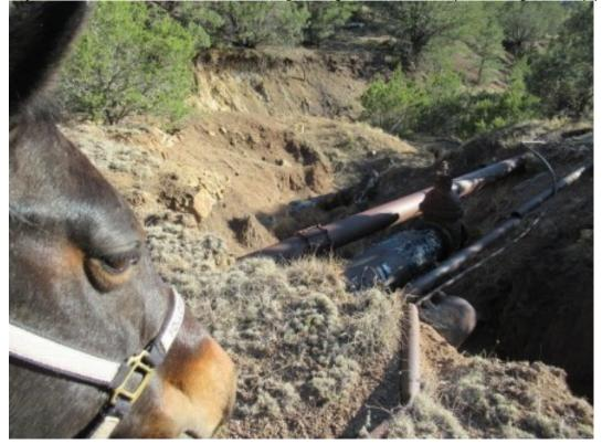
Amazing that these have survived, untouched all these years. Under the more recent metal pipe can be seen remains the original 1907 wood pipe, with its metal wire wrapping. It could carry seven cubic feet per second - about a million gallons a day!
